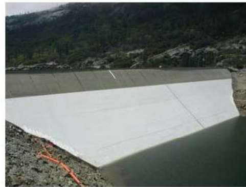
Figure 4: The geomembrane installation at Salt Springs completed with a protection layer installed at the abutments and the reservoir rising in May 2005.
