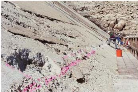
Figure 1: Typical section of the concrete face at Salt Springs dam after 70 years of service and repairs. The shotcrete overlay repairs can be seen in the background.
