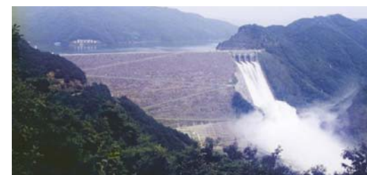
Spillway Discharge in 1990
