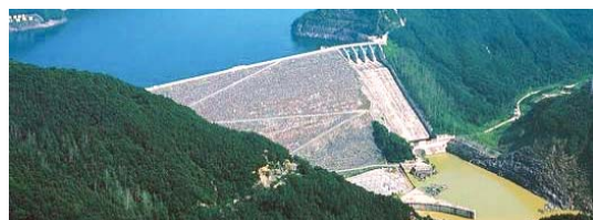
Soyang-Gang Dam as completed in 1973
