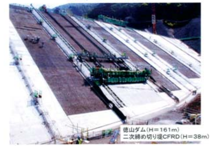
Photo_5 CFRD Dam Coffor Dam of Tokuyama Dam
