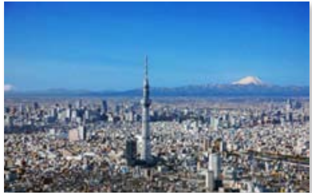
TOKYO SKYTREE® Height=634 m The tallest free-standing broadcasting tower in the world
