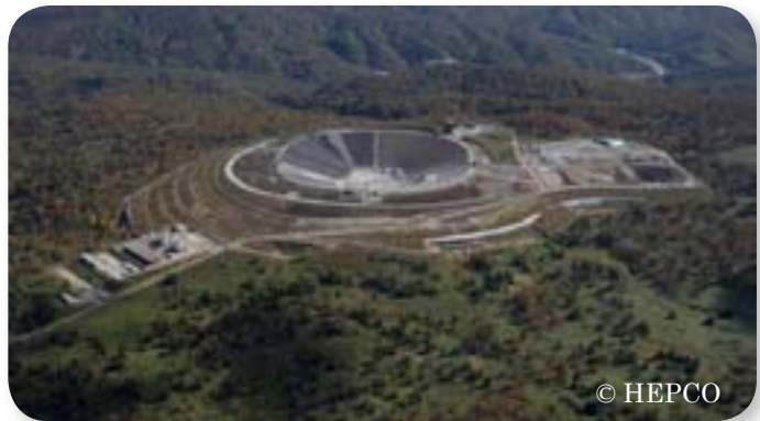
Kyogoku Pumped Storage Power Station Upper Reservoir (Lockfill Dam with Asphalt Facing)
