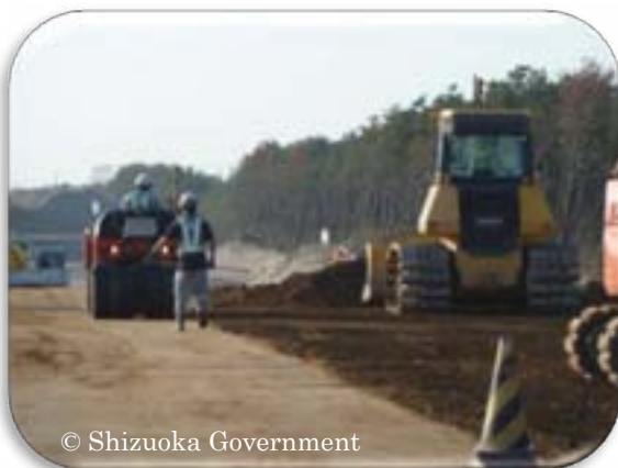
Coastal Levee of Hamamatsu district (Shizuoka Pref.) using CSG Method
