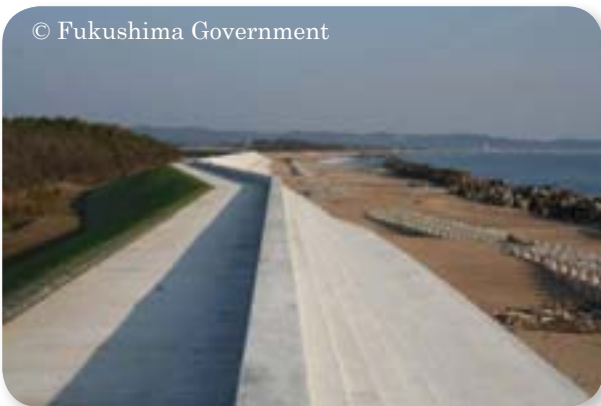
Coastal Levee of Natsui district (Fukushima Pref.) using CSG Method
