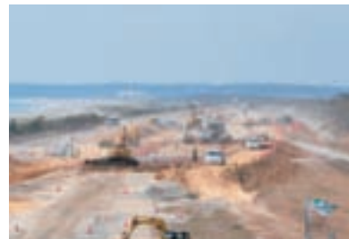
Coastal Levee of Hamamatsu & Natsui district using CSG Method
