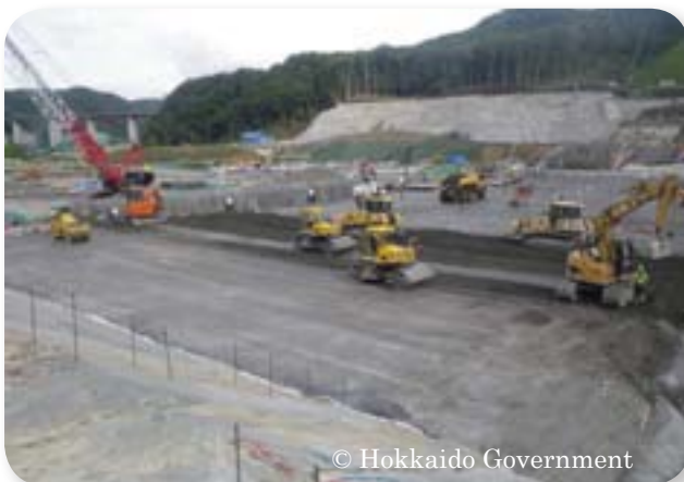
Apporo Dam CSG Placement
