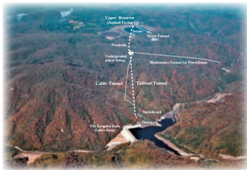
Panoramic View of the Kyogoku Pumped Storage P/S
