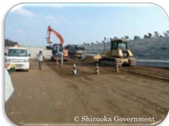
Coastal Levee of Hamamatsu district (Shizuoka Pref.) using CSG Method
