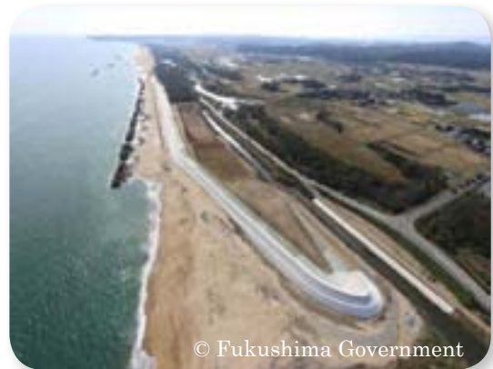
Coastal Levee of Natsui district (Fukushima Pref.) using CSG Method
